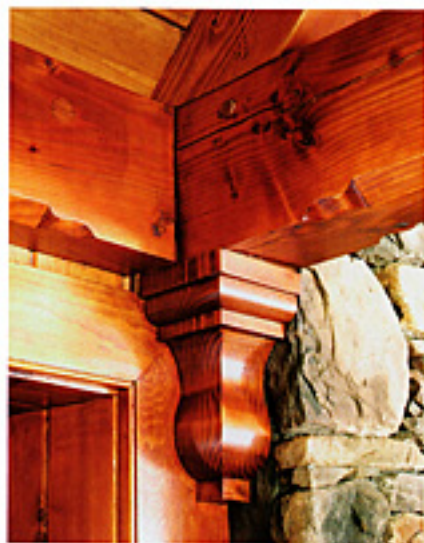
TOP Butternut paneling in master bath fabricated and installed by Stark Mountain Woodworking of Vermont. ABOVE Ceiling beams are Douglas fir with authentic mortise and tenon joints by Olson Development.
