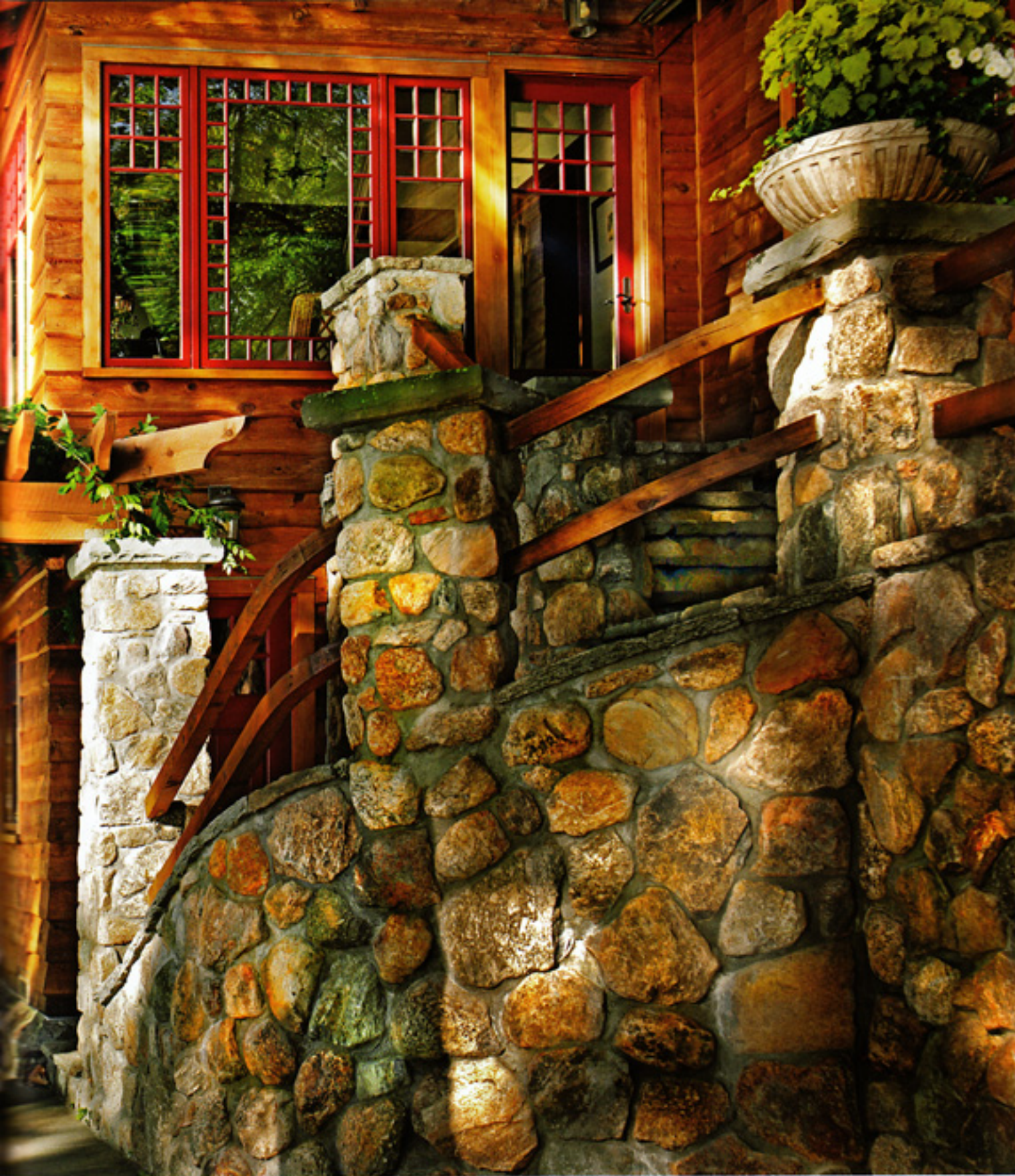
ABOVE Stone native to Connecticut was sensitively incorporated into the exterior walls and patio.
